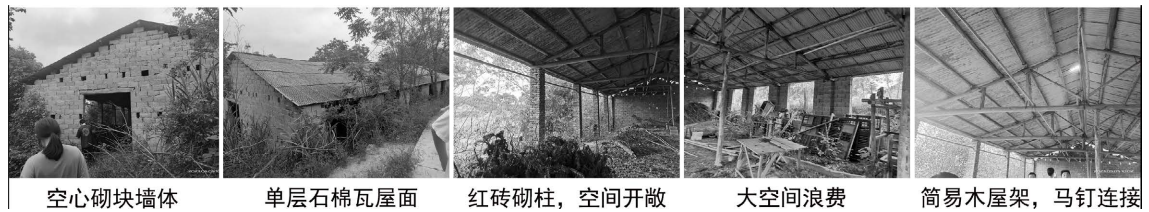
Figure 5. Photographs of the current state of the farm 图 5. 养殖场现状照片
