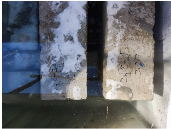
Figure 3. Sulfate-impregnated form 图 3. 试验梁受硫酸盐浸泡过后的形态
