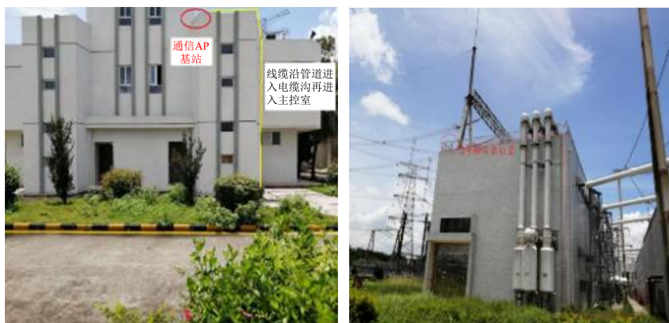
Figure 6. Robot communication AP distribution point position
