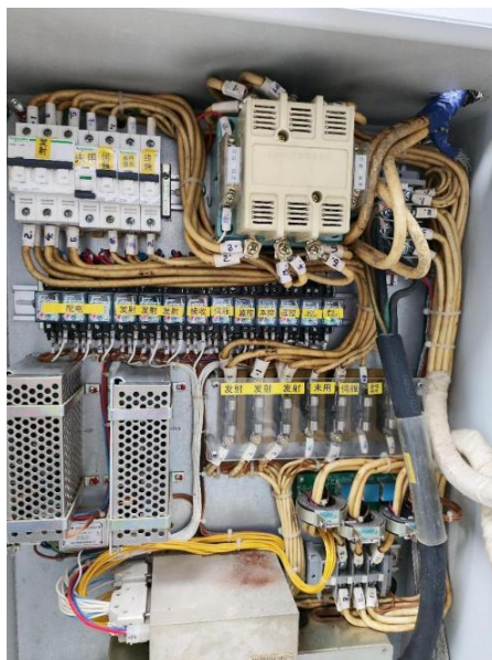
Figure 4. Aging phenomenon of AC contactor 图 4. 交流接触器老化现象图
