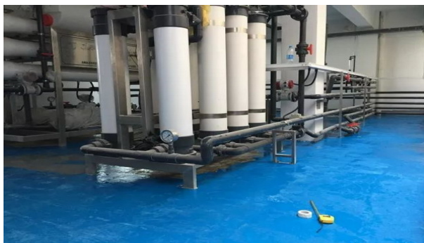
Figure 2. Successful operation of reverse osmosis unit of seawater desalination and utilization system on Lantau Island, Pingtan, Fujian, China 图 2. 福建平潭大屿岛海水淡化利用系统反渗透装置成功运行
