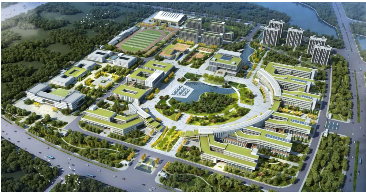
Figure 1. Aerial view of the building
