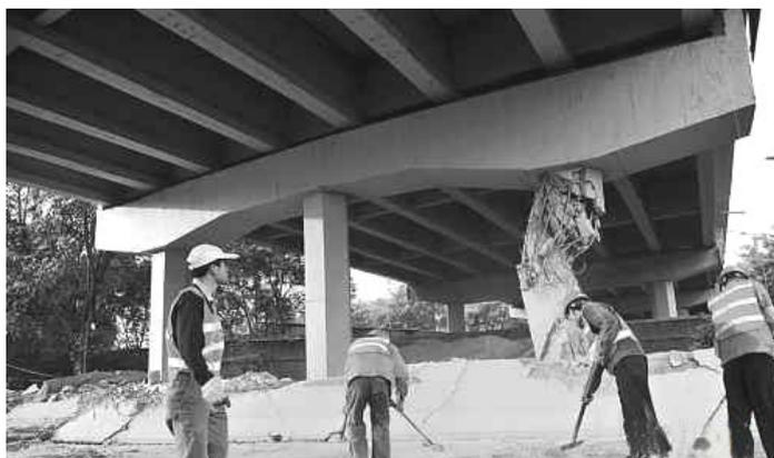
Figure 1. A damaged pier impacted by a flat car
