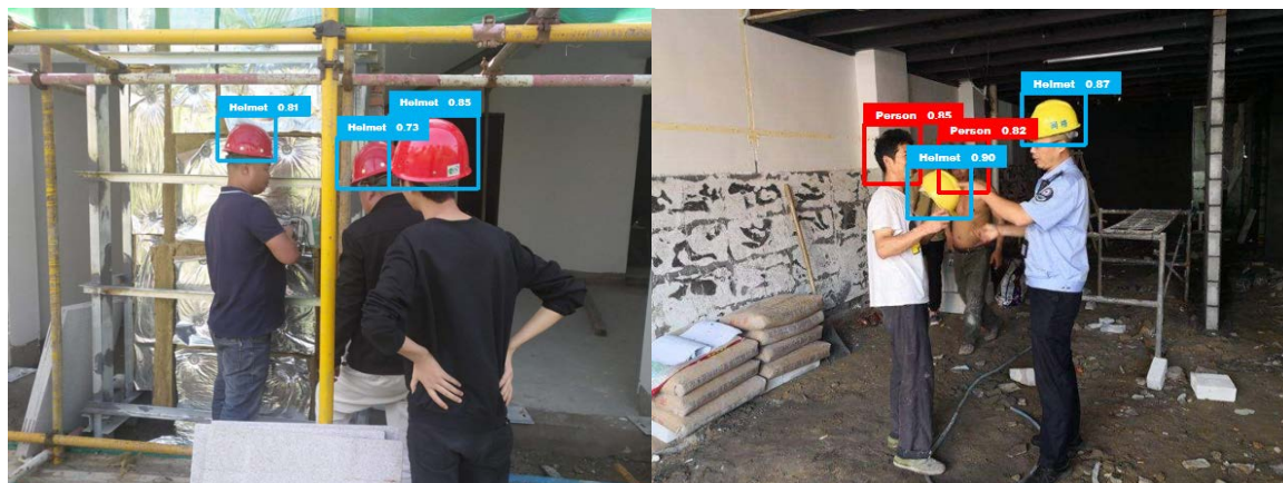
Figure 8. Recognition effectiveness of wearing safety helmets 图 8. 是否规范佩戴安全帽的识别效果
