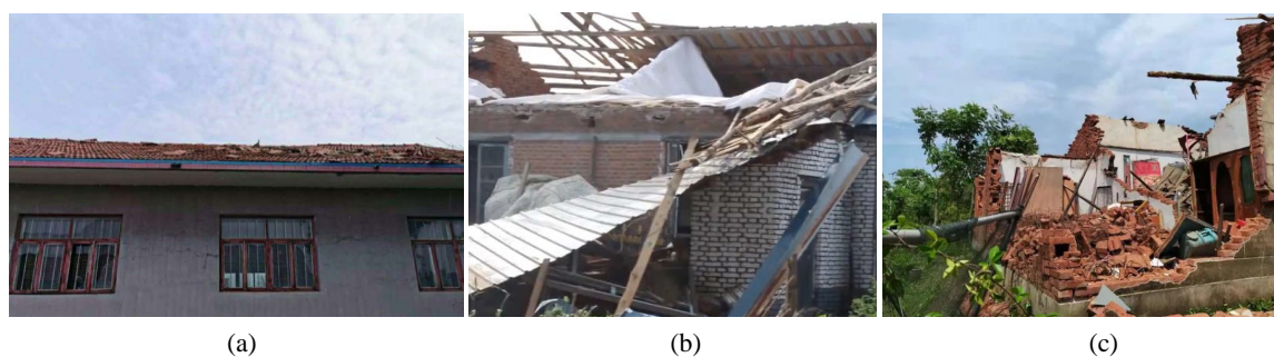
Figure 6. Examples of damaged buildings after tornadoes: (a) Generally damaged (2020.5.18, Weifang, Shandong); (b) Seriously damaged (2017.8.21, Nenjiang, Heilongjiang); (c) Collapsed (2021.5.14, Caidian, Wuhan)
