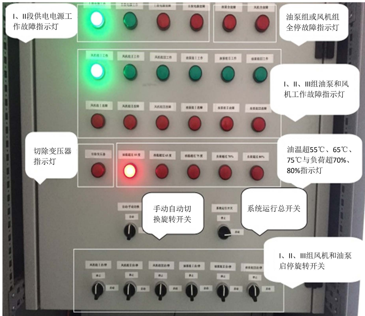
Figure 2. The display and control panel of intelligent control cabinet 图 2. 智能控制柜显示控制面板
