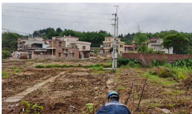
Figure 9. Repair construction of grounding grid 图 9. 台架接地电网修复施工
