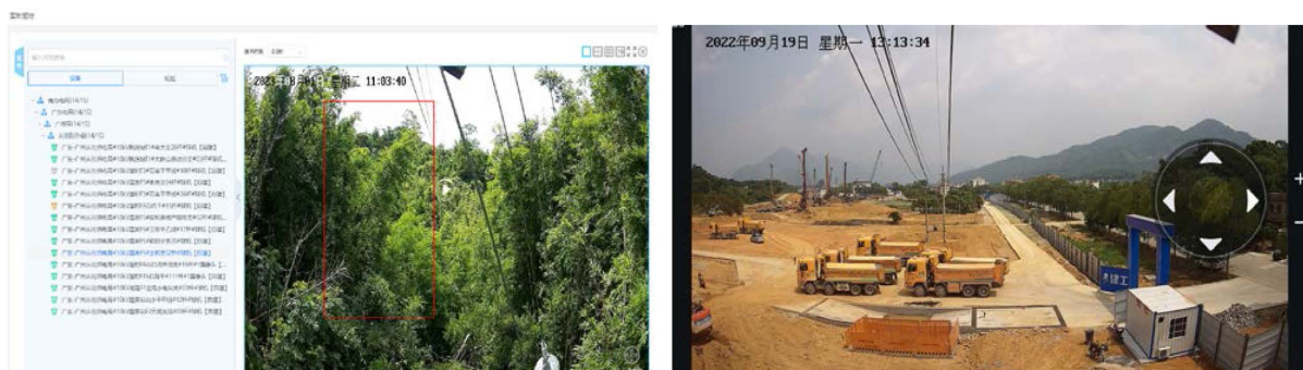
Figure 5. Installation of anti-external damage video monitoring
