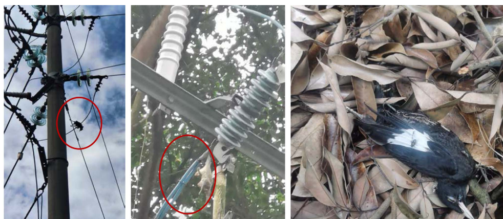
Figure 2. Feeder switch trip caused by small animal touch 图 2. 小动物触碰导致的馈线开关跳闸
