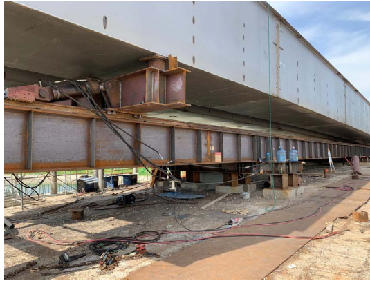
Figure 1. Photo of the nose-deck and guide beam for incremental launching
