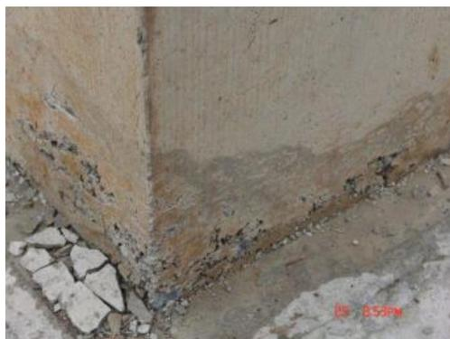
Figure 2. Honeycomb and pitted surface
