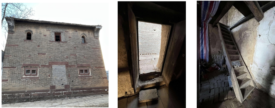
Figure 6. Escape door and stairs of the main house (photographed by the author)
