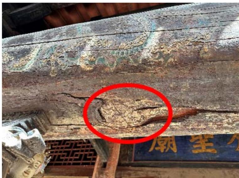
**Figure 3.** Node scars on artemisia wood beams at Cangjie Temple**图 3.** 仓颉庙蒿木檩条的节疤<sup>①</sup>
