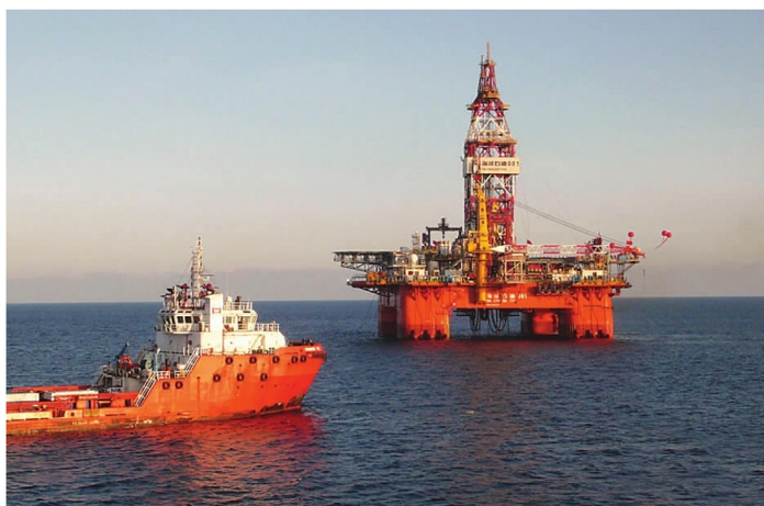
(3) 深水钻井平台 Deepwater drilling platforms
